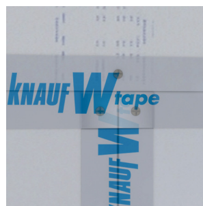
Minst 15 mm underlapp (max 25 mm).
